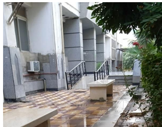
7. Example of Stairs and slope
